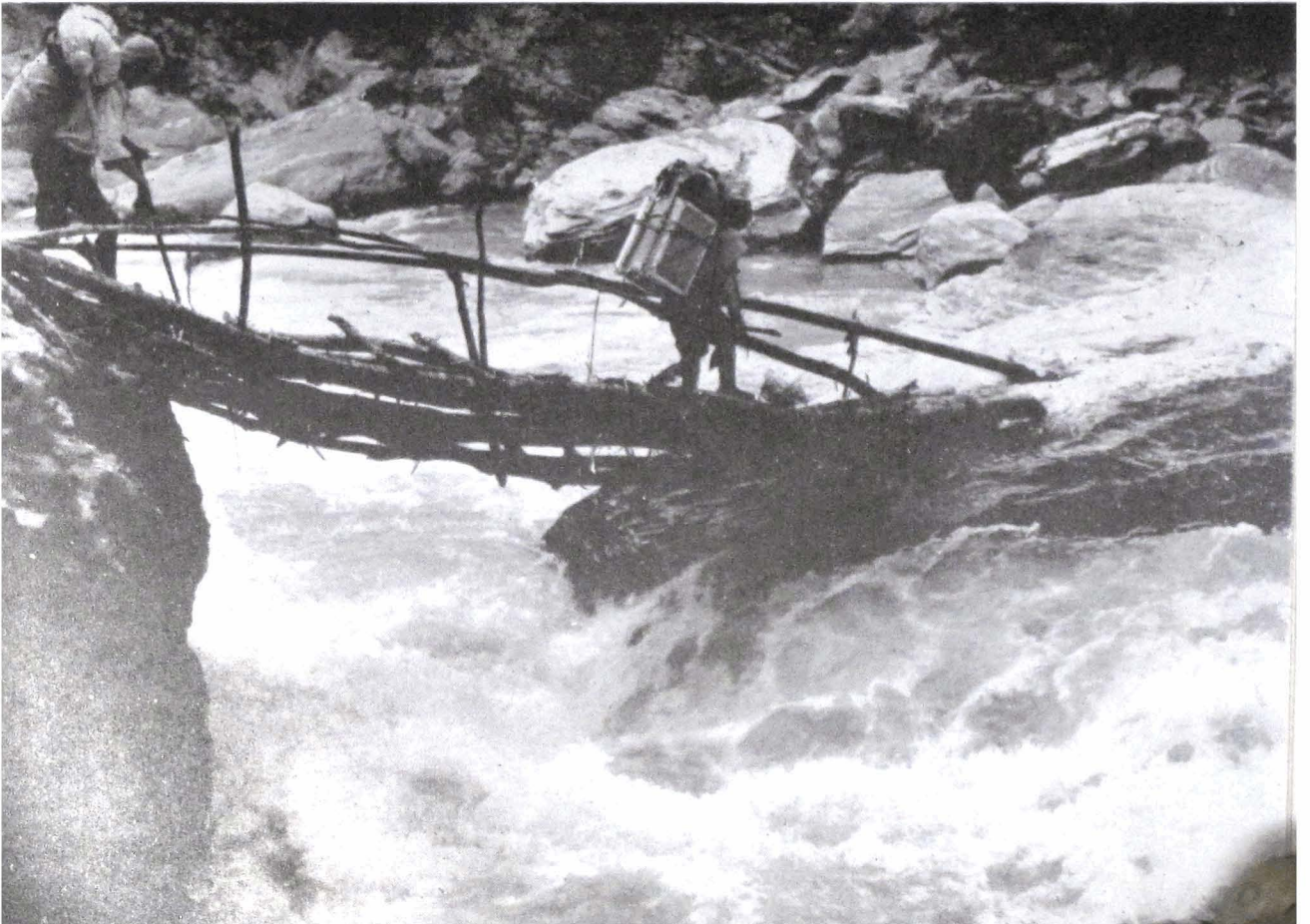
A dangerous bridge across the Dudh Kosi which caused much prayer from the porters as they went over
